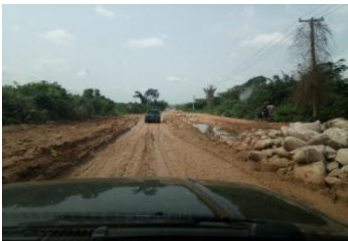
Plate 5.15: Devastating state of the major road
