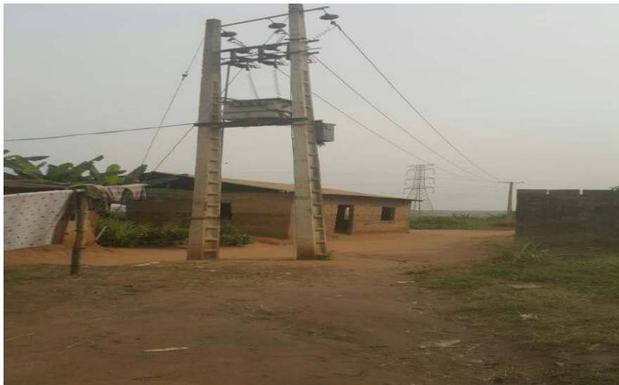
Plate 5.11: Electricity line and Transformer at Soderu Community
